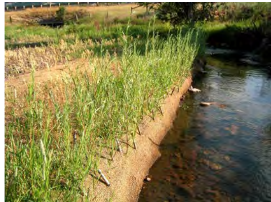
Willow cuttings work well planted through geotextile fabric if the basal end of the cutting can reach the water table. Irrigation is also useful to help establish new cuttings.
